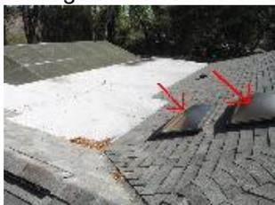
*ADDITIONAL COMMENTS:* Garage skylights show old water damage. Tested, no active moisture at the time of inspection.
