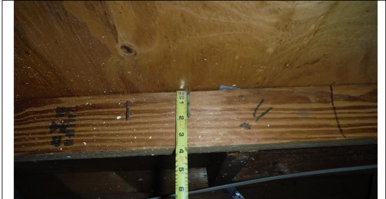
8 D nail decking attachment.
