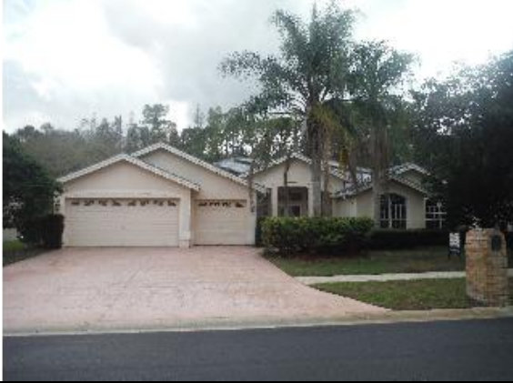
Front of structure
