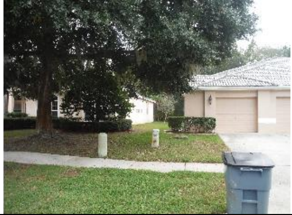
Right Side of structure
